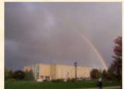
SWRZ Building Purdue North Central
